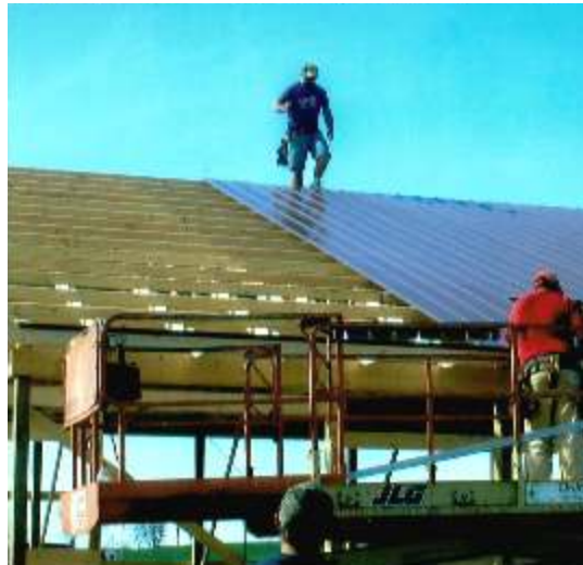
Workers install the roof on the new office building. submitted
