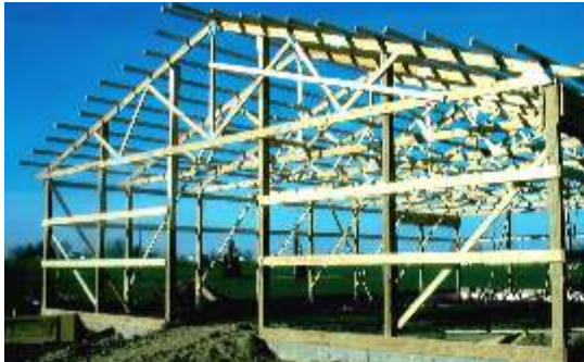
Construction began on the new Festival office building. submitted
