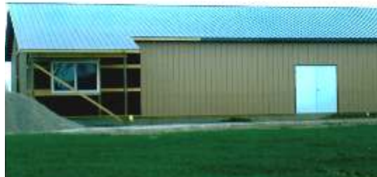
This photo shows the current Sweet Corn Festival office building nearing completion 12 years ago at historic Lions Park. submitted
